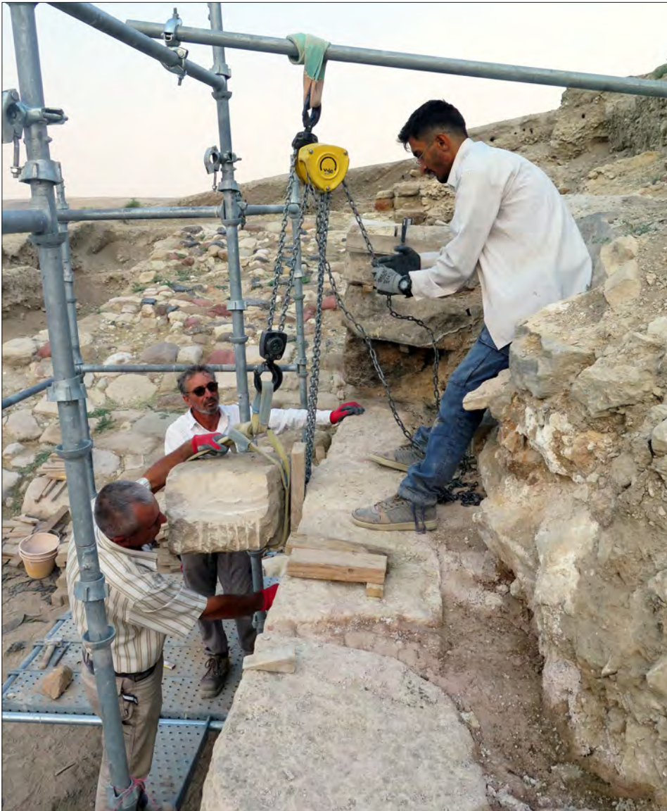
Figure 8: Nahit Yılmaz, Angelo Lanza, and Alican Kircaali moving a conserved wall stone back into its original position on the South Gate. Photo by Elisa del Bono.
