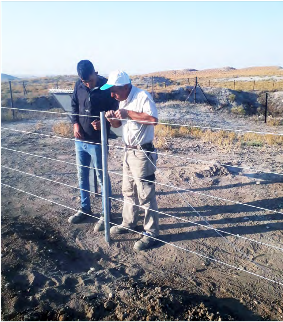
Figure 12: Installing the new galvanized fencing on Gordion's visitor circuit. Photo by Ömür Atıktığ.
