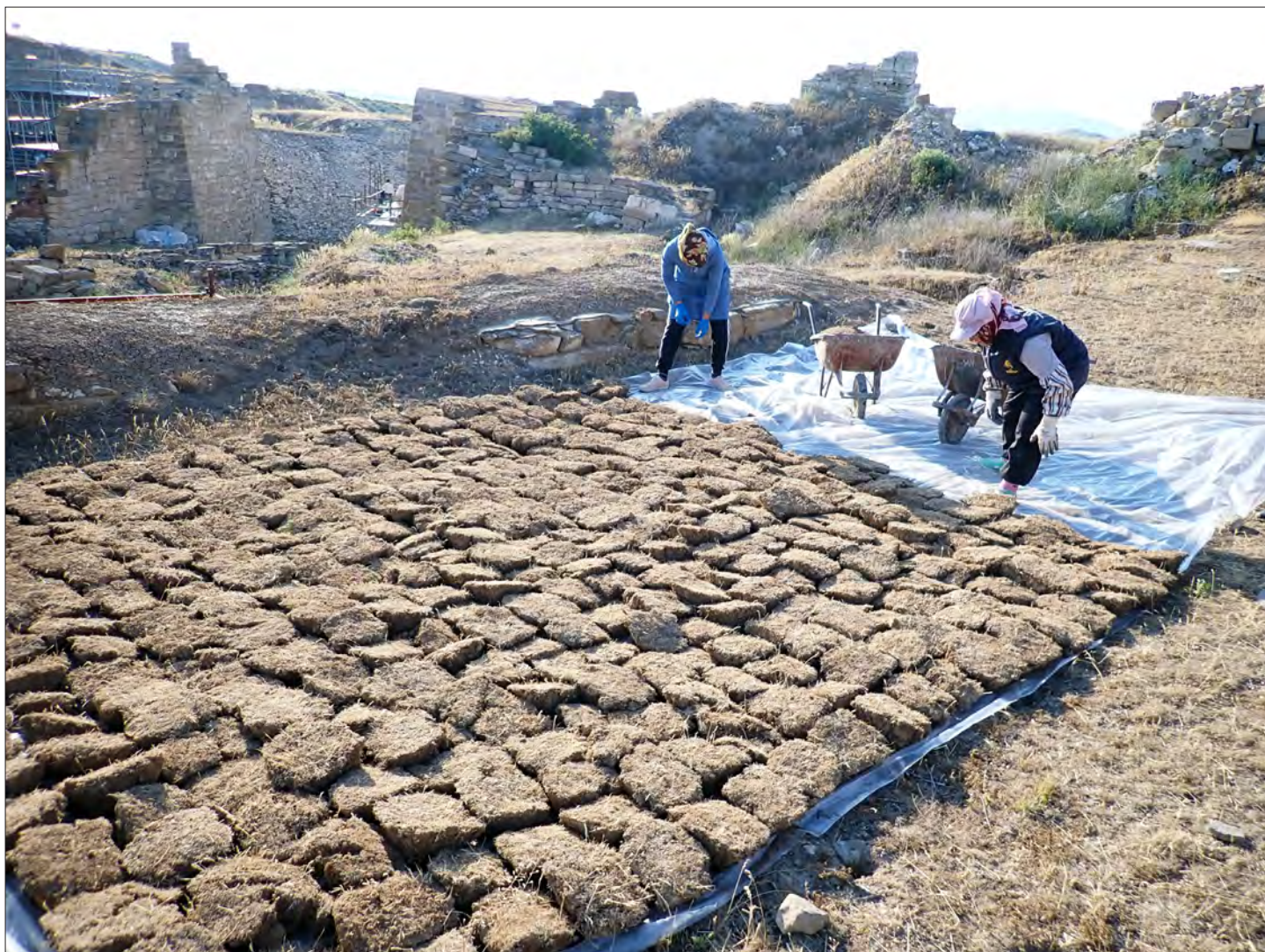
Figure 13: Preparing the “green caps” to be placed above the conserved walls of the 9th century B.C. Terrace Building. Photo by Brian Rose.
